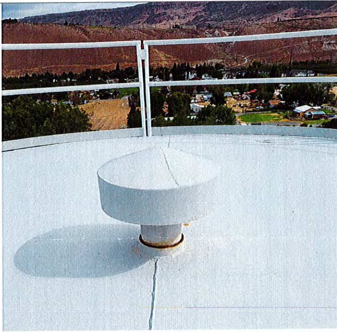
Reservoir roof vent
