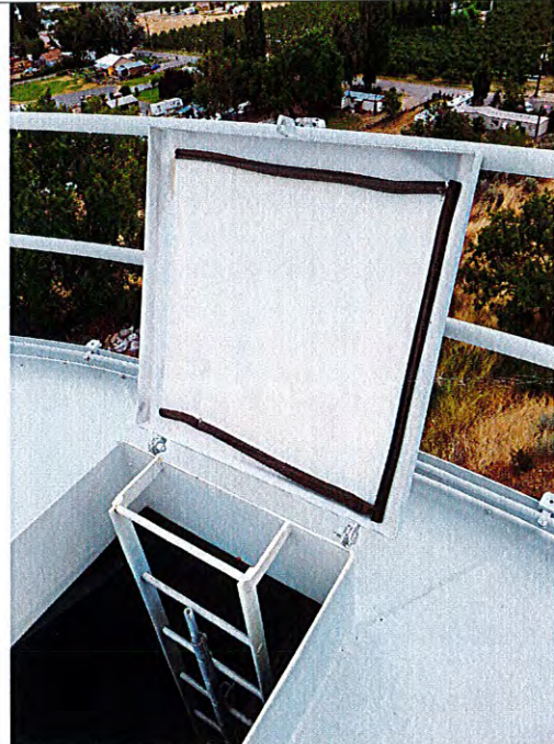
Reservoir access hatch – gasket material in the lid needs to be replaced such that the seal between the lid and curb makes is watertight.
