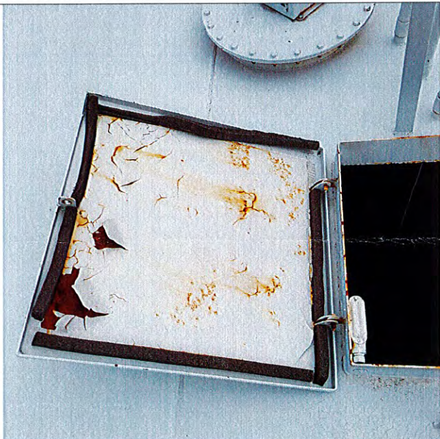
Reservoir access hatch – gasket material in the lid needs to be replaced such that the seal between the lid and curb makes is watertight.
