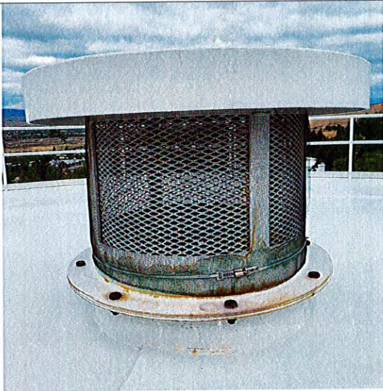
Reservoir roof vent
